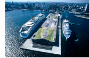
Osanbashi Yokohama International Passenger Terminal
