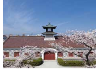
旧新潟税関庁舎 Former Niigata Customs House
