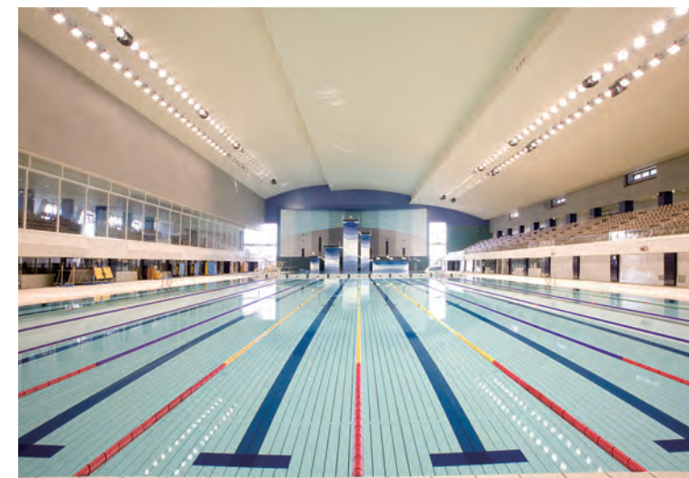
The 50m pool can be split up into two 25m pools for different uses. (Moving floor)
