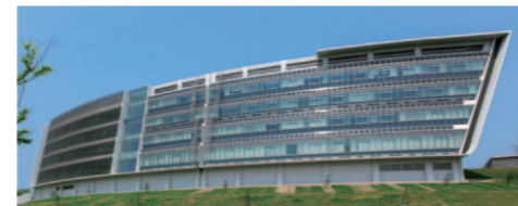
External appearance of buildings (the left part from center: I2CNER, the right part: NEXT-FC)
